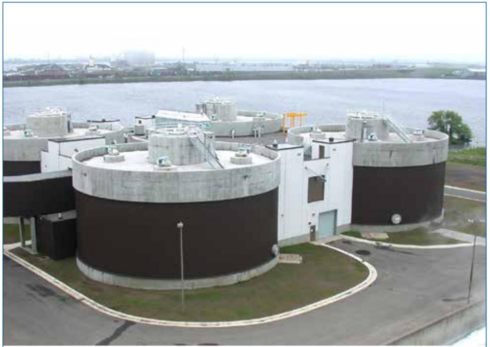
**These four large tanks are the anaerobic digesters that produce Field Green® biosolids. Anaerobic, or oxygen-free, digestion uses bacteria to produce biosolids and methane. The methane is burned to produce heat and electricity.**
