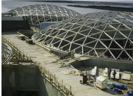
WLSST construction (April 1978)
