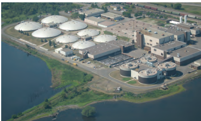
WLSST's wastewater treatment plant today
