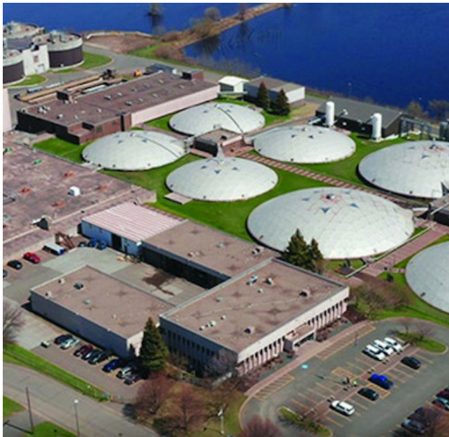
Western Lake Superior Wastewater Facility
